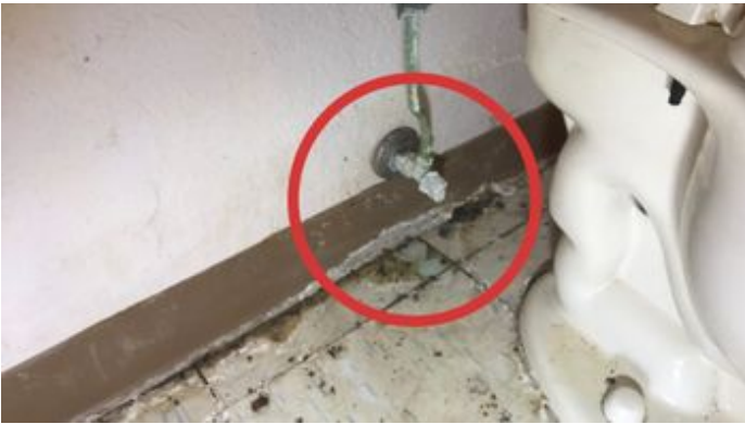
Leaking toilet valve. Located at garage bathroom in main home
