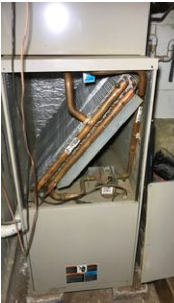
Forced air Water furnace system. This appears to be disconnected or possibly abandon. It was not operational during the inspection.
