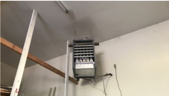
Heat exchanger located in additional garage. This unit appeared to be shut off and not operational using normal operating controls during The inspection. Recommending licensed HVAC technician further review.
