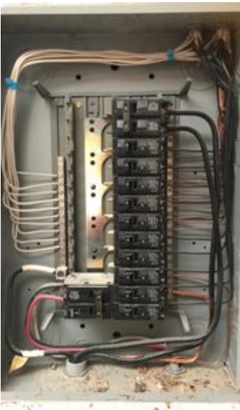
100 amp sub panel located at interior
